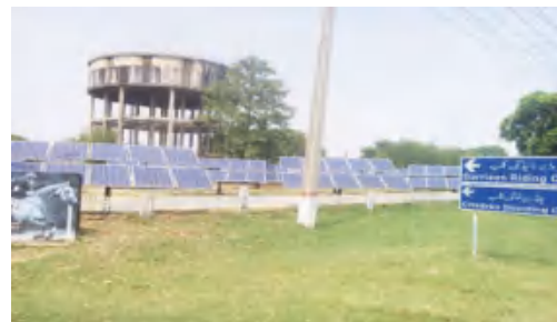
System: 22kw system Application: Agriculture Irrigation Location: Gilgit Baltistan Province, Pakistan Head: 160feet
