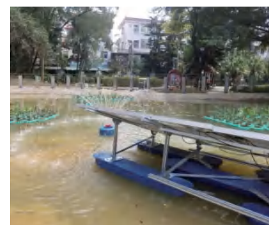
System: 2 sets 750W solar aeration system Location: Shenzhen
