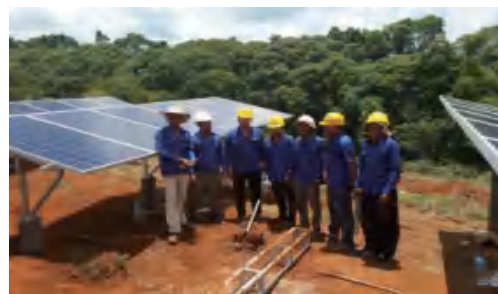
System: 4KW Solar Pump System
