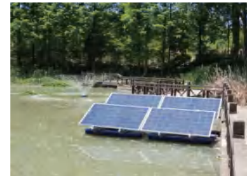
System: 1.1kW solar aeration system Location: Hefei
