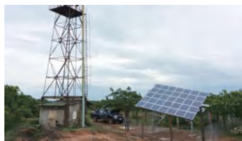
System: 3.7kw solar pump system Location: Cambodia
