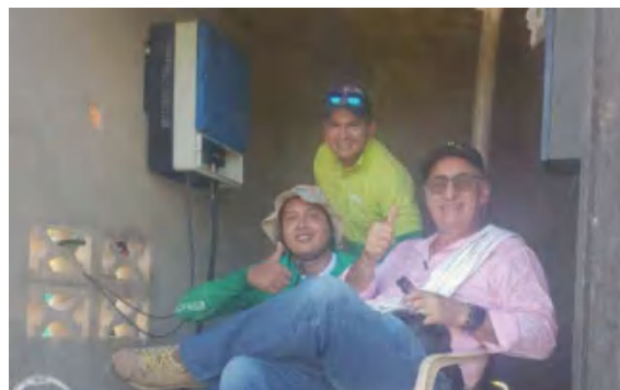
System Solution: 18.5kw system Application: Agriculture Irrigation Location: Colombia
