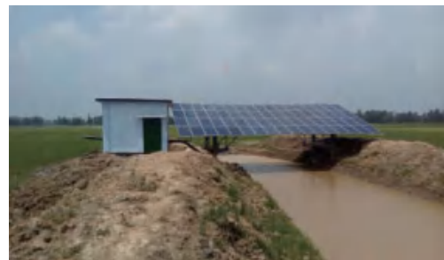
System: 2.2KW System Application: Agriculture Irrigation
